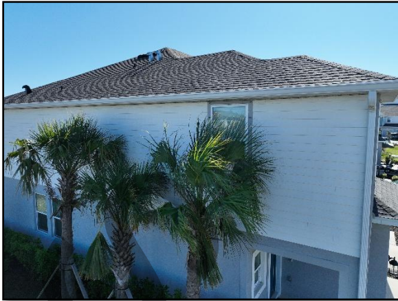
92 - Landscape touching building / structure / wall. M19_UAV(1701)
