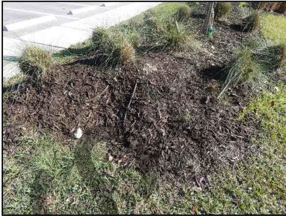
86 - Exposed drip lines and bubblers. M08_(2303)
