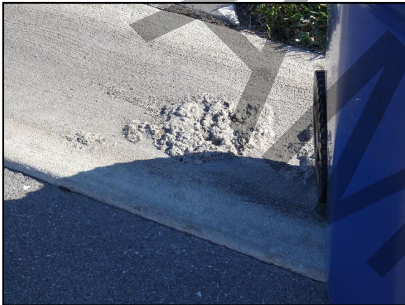
50 - Concrete in gutter. M57_(155)
